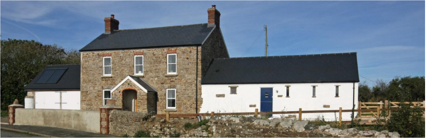
Glebe House - sleeps up to 10 and only a mile from the beach and 200 yards from the Coastal Path
